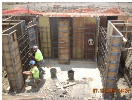
Figure 4: Mod-U-Form installation
