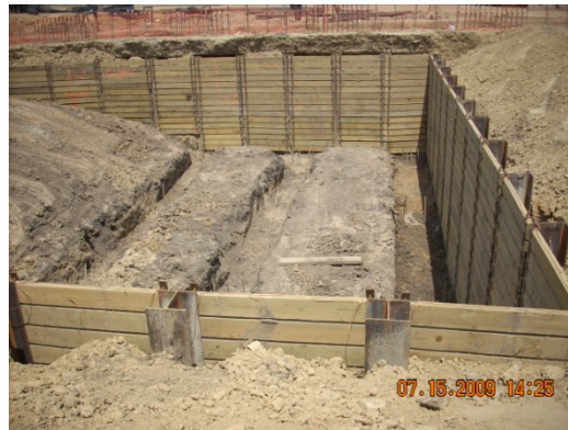
Figure 6: Supported excavation around pool
